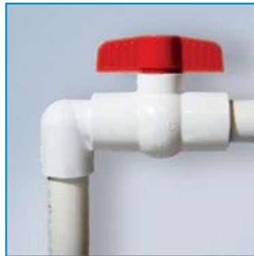
1" Fresh Water Tank Drain
